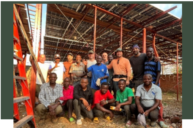
The Team completing the installation of 72 solar panels.
