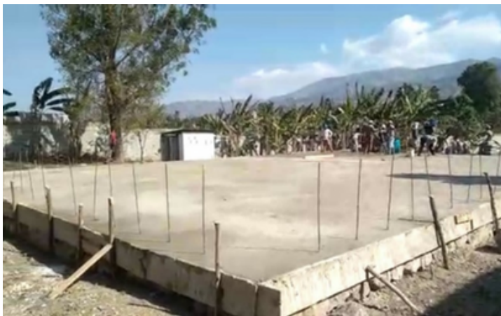
Completed Susanna Wesley Clinic foundation, building for the future.
