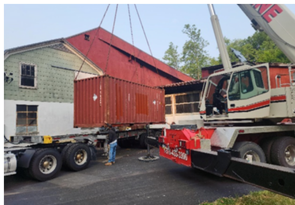
The container with solar components and medical equipment loading in Montoursville PA
